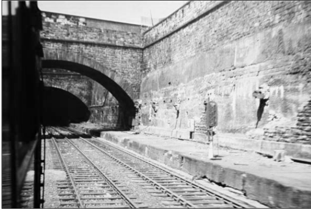
The remains of St. James' Station in 1968. Taken from a Down train, the view shows the out of use middle road from Liverpool Central to Brunswick, the Up line and former platform and the rear of Brunswick's Up Outer Home signal (No. 51).
