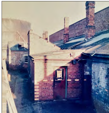
Above : Taken in 1987, immediately prior to the demolition of the MPD, this photograph shows the particularly unimposing entrance to the depot.
