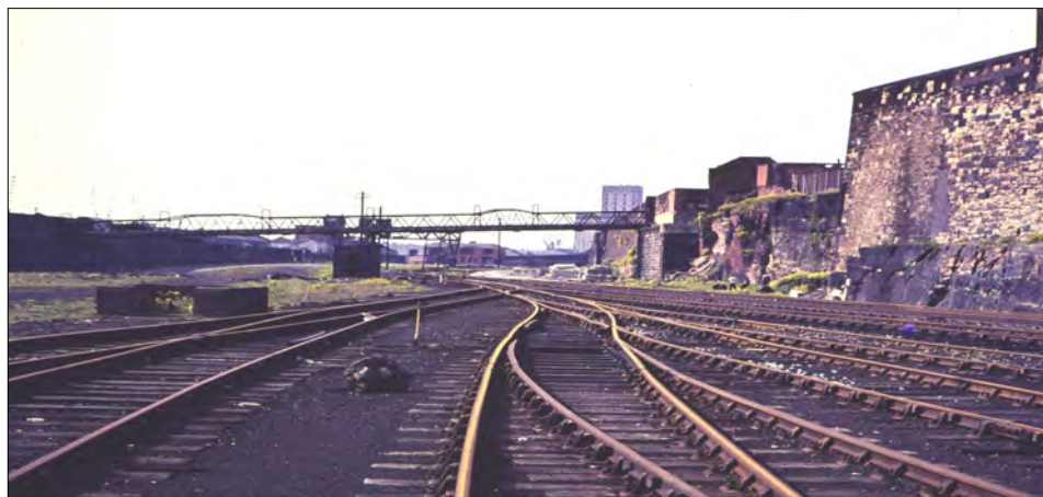
Above : Looking towards Liverpool, the site of Brunswick Signalbox and the site of the new passenger station; as seen in the dying weeks of the oil trains, and 18 months before electric trains started to pass the site - 16 May 1976.
