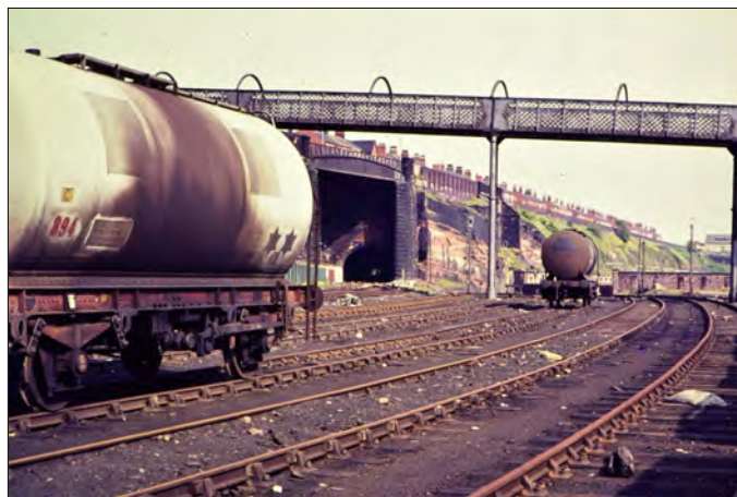
Above : Brunswick Yard on 16 May 1976 – the work on the Down line in Dingle Tunnel can be seen.
