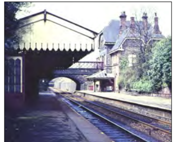
Above : The cramped site of Cressington station, sandwiched between two road overbridges. Dispensation on minimum platform width requirements was needed to extend the platforms under the northern-most bridge and into the cutting after the station reopened.
