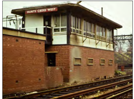
Above : Hunts Cross West Junction box in early 1983 – decommissioned and awaiting demolition.
