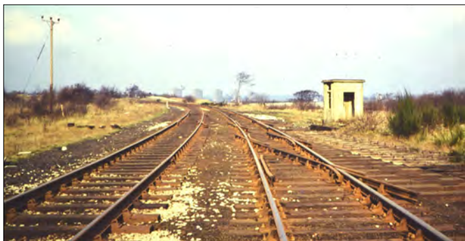
The site of Halewood North Junction in 1971
