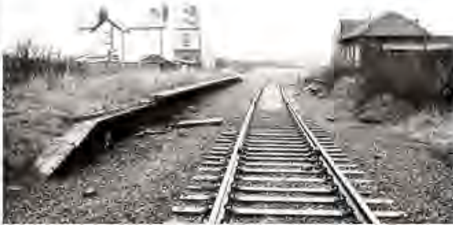
Appleton Station as seen looking south in January 1962. The last trains had run through the station in November 1961. The line through the station had been singled at the end of 1973. John Mann
