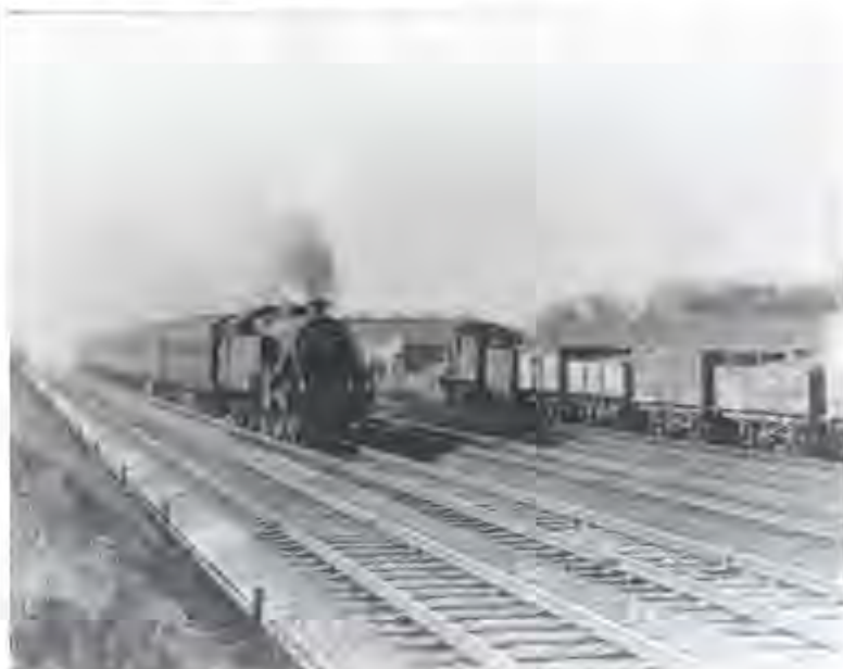
Looking west on the 28 th of March 1959 as a Manchester Central service passes the sidings that were situated adjacent to the CLC main line within the 'Halewood Triangle'. Jim Peden
