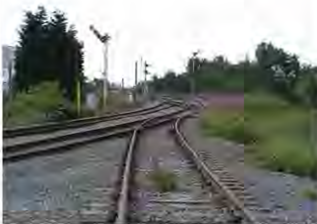
Looking west at the junction between the deviation and the yard at Tanhouse Lane in July 2005. P Wright
