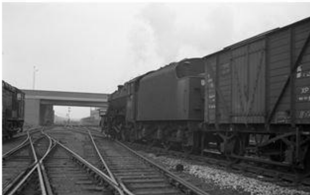
Another 8F this time on a train of vans heads west towards Widnes West Deviation Junction. To the left can be seen a 350hp Shunter (Later class 08) which would have been one of the trip locomotives that was based at Hutchinson Street Yard. – Photo by Les Fifoot.
