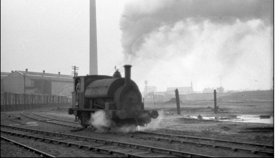
'Lucy' at Hutchinson Street sidings in February 1968. This was the location at which the Widnes Dock Estate railway connected to the Garston and Warrington line. Waggon's would be marshalled at this point and then taken away by British Railways locomotives.
