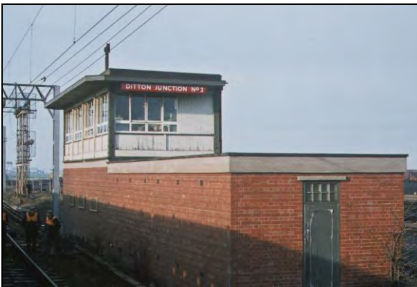
Ditton Junction Number 2 Signal Box. Photo by Ken Booth.
