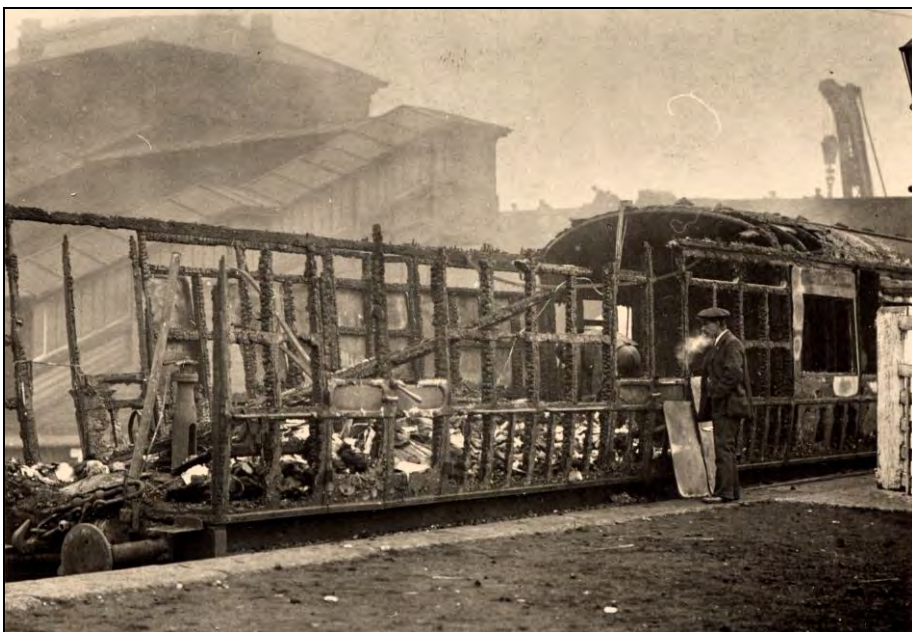
A burnt out coach from the ill-fated 5.30pm Chester to Liverpool service. The coach is seen standing at Ditton Junctions goods platform. The present day signalbox which opened in 2000 now stands at this location.
