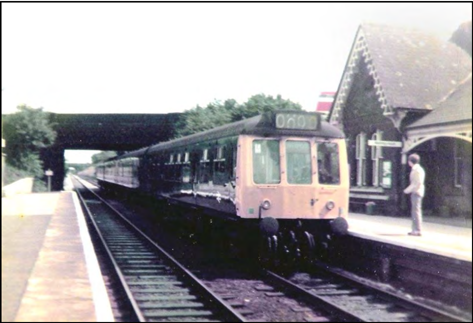
Widnes station (latterly Widnes North) in the summer of 1977. Photo by Paul Wright
