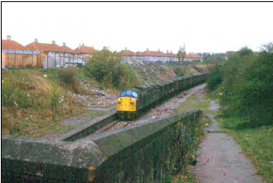
Looking north down the southbound platform access ramp at Knotty Ash station in the early months of 1975. A class 40 locomotive on the 9T21 working from Huskisson Dock to Edge Hill can be seen passing through the station. Photo by Norman Daley
