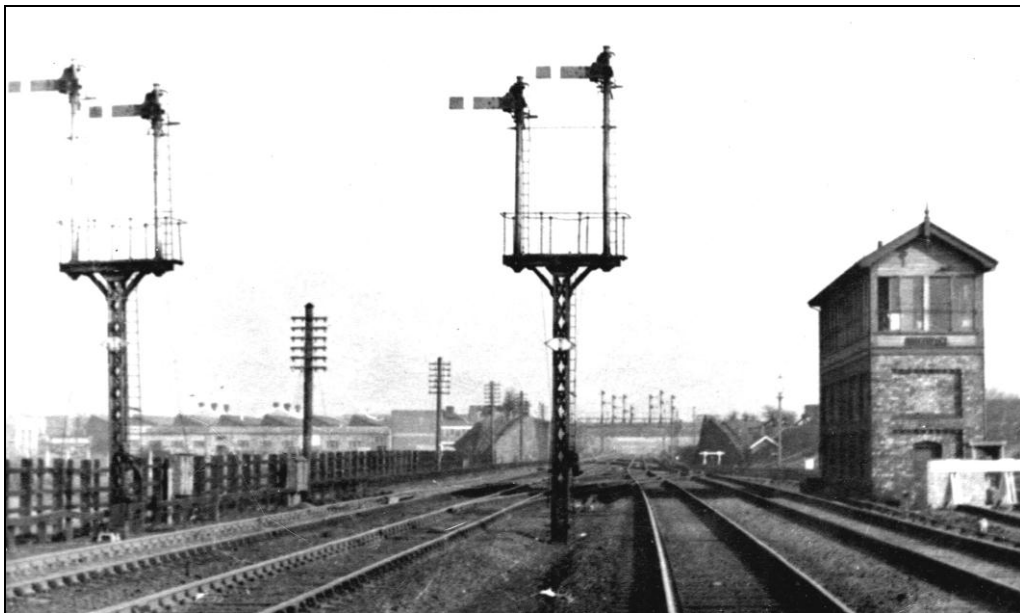
Looking east at Speke Junction in the 1950s along the up slow line. This would be the view seen by the driver of the London Express Goods train fired by Barry Nolan in 1958. The Ditton troughs lay only a few miles distant. Photo from the Richard Mercer Collection
