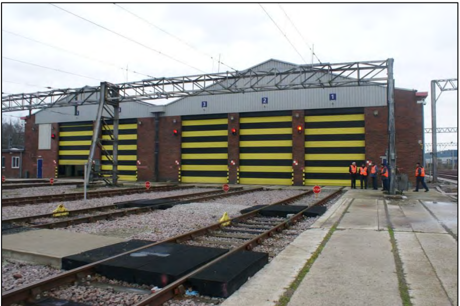
The depot building at Allerton looking east on 14 December 2013. The clean and tidy appearance of the depot is a credit to the Northern rail staff who work there. Their depot had probably not looked so good since it opened in 1960. Photo by Paul Wright
