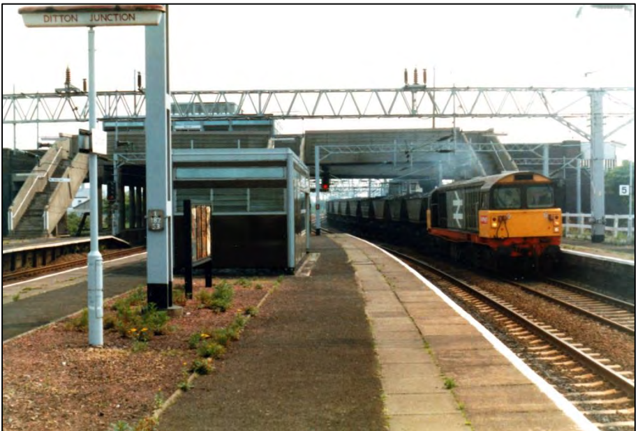
Ditton station looking east along platform 4 on 11 May 1987. Class 58 locomotive number 58 018 is seen passing through on the down slow line with a Toton to Garston working. Although the station had been renamed as Ditton in 1973 the lamps still carried the name Ditton Junction. Photo by Terry Callaghan
