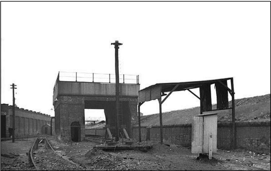
The coaling facility at Widnes Shed seen on 7 August 1964 after the shed had closed. Due to its cramped location every inch of space had to be put to productive use. Photo by Alan Robinson
