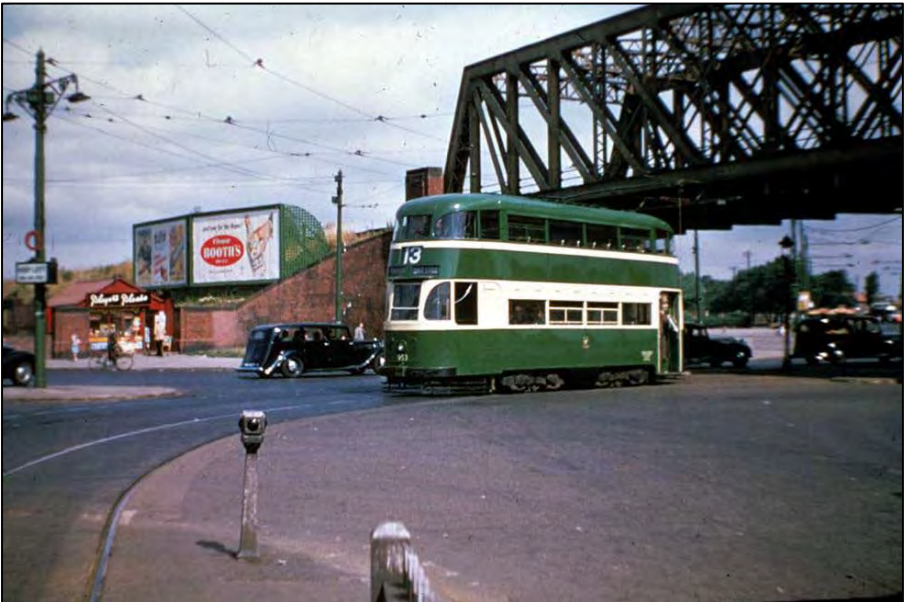
A Liverpool bogie steamliner is seen passing under the CLC Halewood – Aintree line at Clubmoor in the late 1940s. At this location passengers could change between tram and train. There were two types of steamliner the bogie version seen in this view and a four wheel version known as the 'Baby Grand'.
