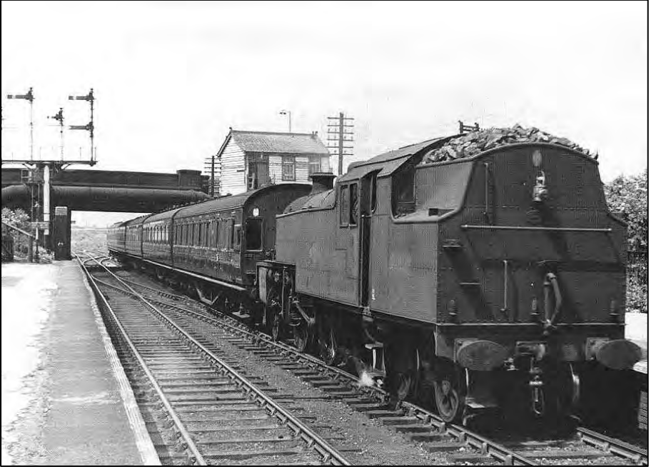
Hindley South station looking north in the early 1960s as a Wigan Central to Manchester Central passenger service arrives. Six coaches were far too generous for the number of passengers who were using the line at the time.
