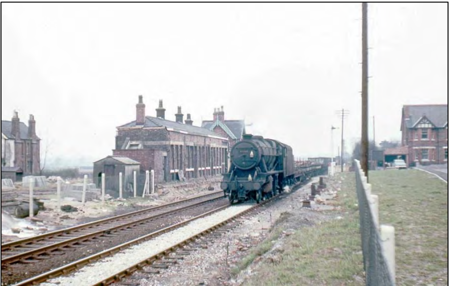
Looking east at Lymm station on 29 March 1968 as a westbound freight passes through. Photo by Bevan Price
