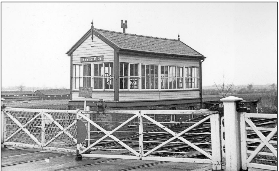
Lymm signal box seen in 1972. It was at this location in the early hours of a Friday morning in 1963 that Dave Littler was informed that a derailment at Northenden had stopped his progress towards Stockport Edgeley. Photo by David Ingram
