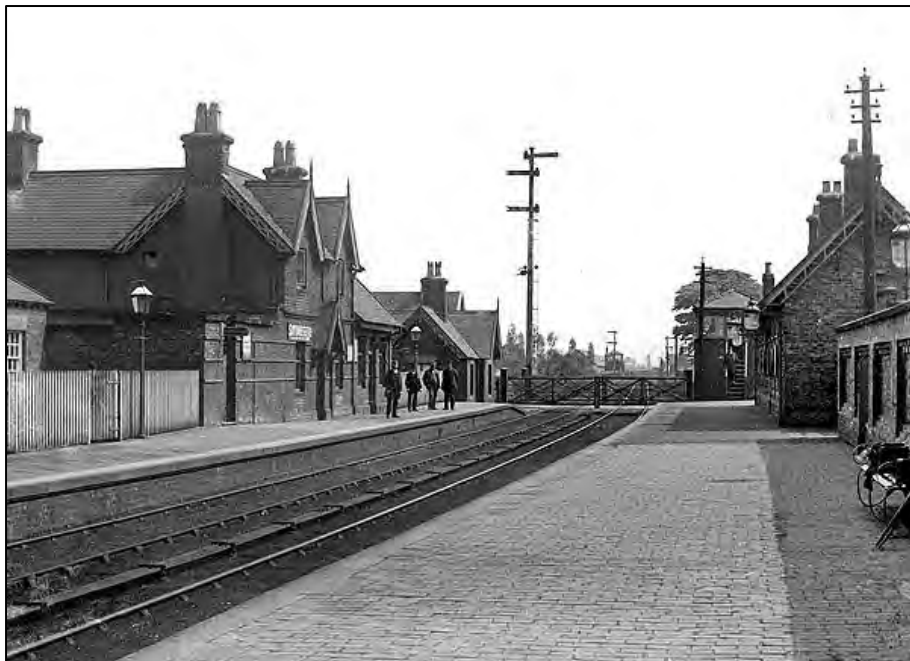
The original Latchford station seen in 1889. The station closed on 10 July 1893 when all traffic was switched to the Latchford viaduct line which had been brought into use for goods services in February 1893.
