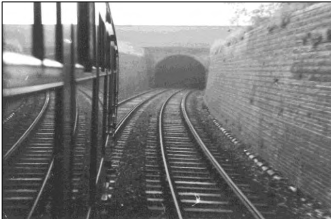
Left – The north portal of the Liverpool Road tunnel seen from an up (Warrington direction) train in 1964.
