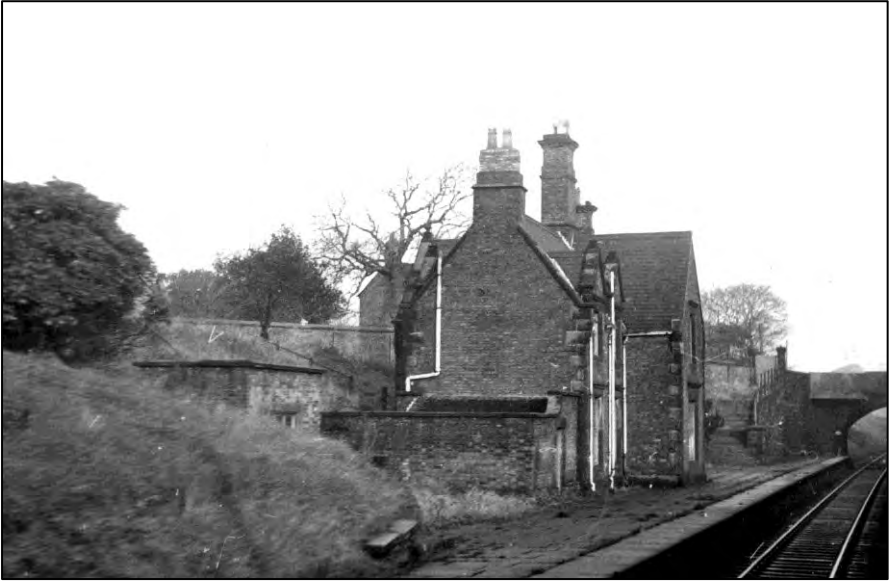
Daresbury station seen from a passing train in the 1960s. The station had closed on 7 th July 1952. Photo by John Kirwood
