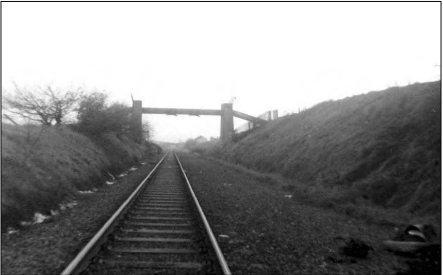
A view from 1981 looking south towards Appleton along the 1850 alignment that replaced the inclined plane at Widnes. The inclined plane would have been to the right of the alignment shown in this view. The line became single at this point with effect from 4 th November 1973. Photo by Paul Wright
