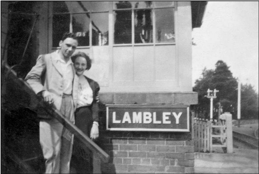
My parents photographed on the steps of Lambley signal box in 1938. The box was located on the station platform.
