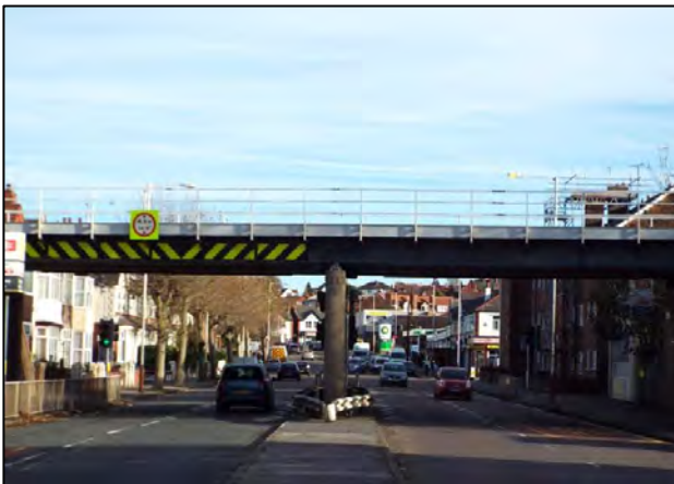
Left: The bridge at Wallasey Village that Eric Smith worked on in 1965. Photo by Rebecca Hicks
