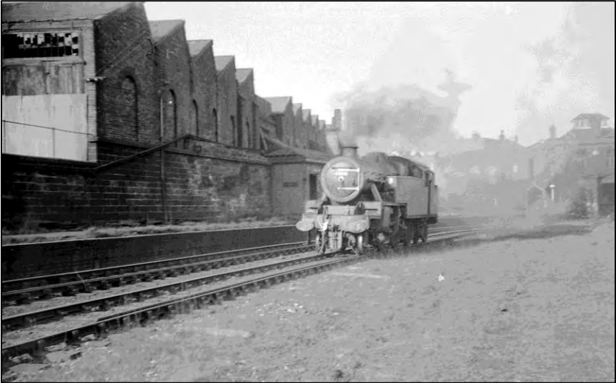
Seen passing through the remains of Birkenhead Town station on 5 March 1967 is Fairburn 4MT 2-6-4T locomotive number 42616. The engine was on its way to Birkenhead Mollington Street shed having worked a train into Birkenhead Woodside station. Photo by Richard Mercer
