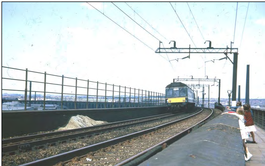
A Liverpool to Chester DMU is seen running wrong line towards Runcorn in 1967. The wrong line working had been introduced due to engineering works. The pedestrian footpath was closed at this time but that does not appear to have stopped local children from gaining access. Photo by Les Fifoot
