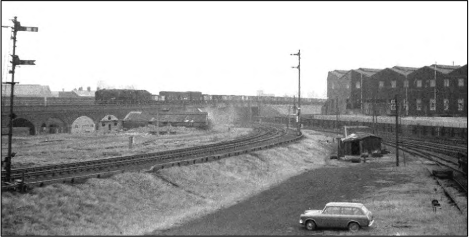
Looking north-east from the pedestrian footbridge at Widnes Dock Junction in August 1967. This location had been a very busy railway location but it was in decline when this view was taken. In the distance a coal train can be seen heading west towards Garston on the Widnes Deviation line. To the left is the Deviation St Helens line spur and to the right the original route to Garston. The car most likely belongs to the signalman who would have been on duty at Widnes Number 4 box. Photo by Alan Robinson
