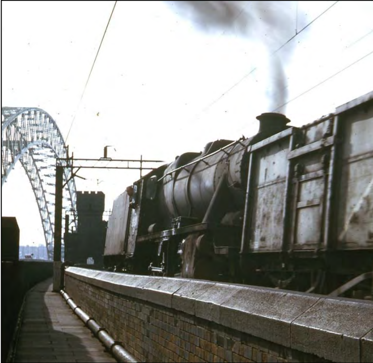
Looking towards Runcorn from the pedestrian footpath as an 8F locomotive heads towards Runcorn with Target 92 in 1967. Photo by Les Fifoot.
