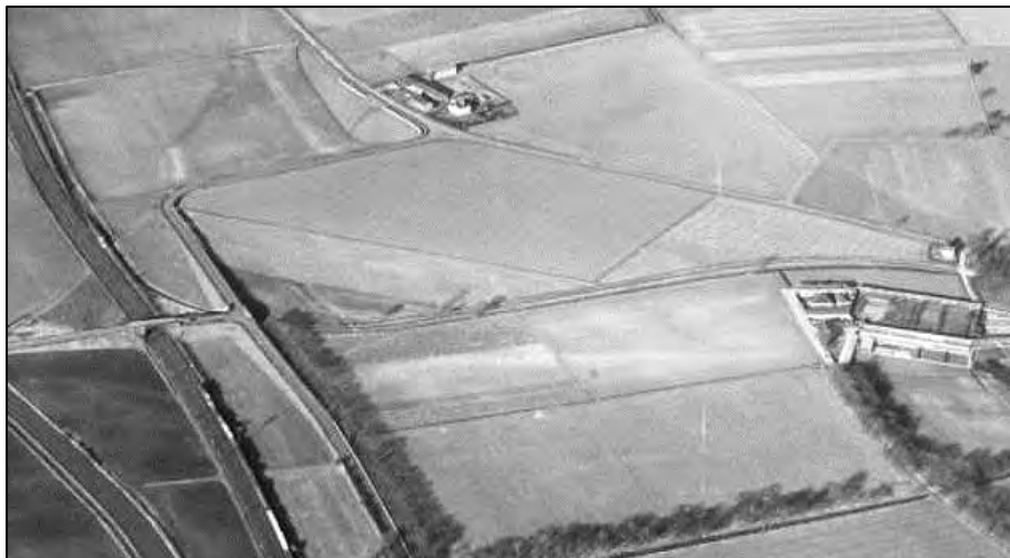
An aerial view showing the western end of the Winwick Hospital Branch as it was in 1947. The main line can be seen to the left with the branch curving off to the right where it passes under Watery Lane.
