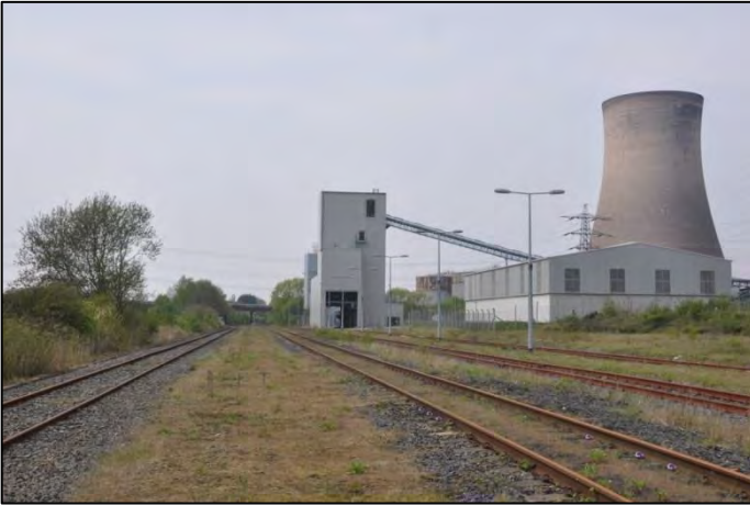
Left: A lack of trains had left the tracks at Fiddlers Ferry Power Station looking rusty when this view was taken on 7 th May 2016. Photo by Doug Birmingham
