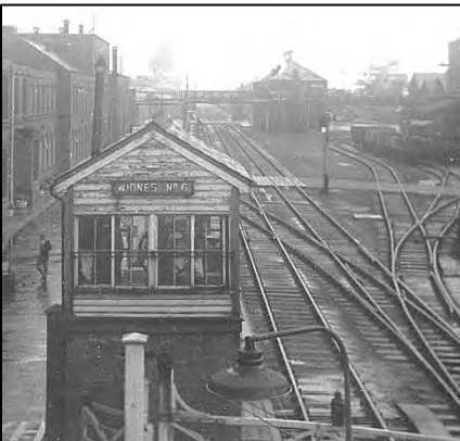
Widnes Number 6 signal box looking east from the Waterloo Crossing footbridge in the early 1960s. Widnes Number 6 was located on the original course of the Garston and Warrington railway which had opened at this point on 1 st July 1852. The original Widnes station (opened as Runcorn Gap) was directly behind the photographer. It was replaced on 1 st March 1870 by a new facility on the Deviation line. The original line through Widnes was then downgraded to a goods route. The section of line seen in this view closed on 10 March 1969.
