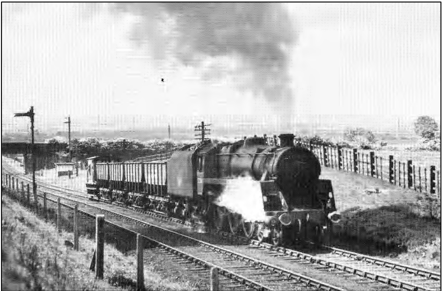
The bank at Chequerbent on the former Bolton & Leigh railway was notorious with locomotive crews and in the winter months fireman had to walk in front of trains shovelling sand and grit under the locomotive wheels as described by Barry Nolan. In this view a short coal train is seen going up the Chequerbent bank.
