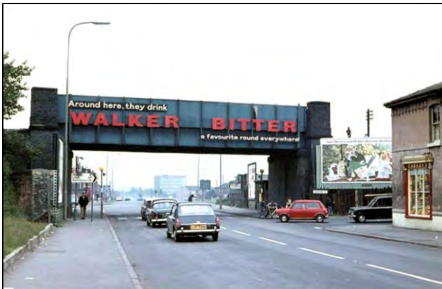
Left: Looking south down Winwick Road towards Warrington in the late 1960s. The Warrington avoiding line is seen passing over the road. Photo from Neil Wilson
