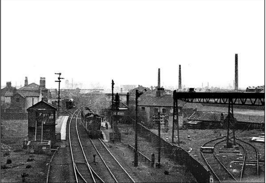
Looking south at Appleton station in 1948. Standing at the up platform is a service for St Helens Shaw Street. This is the station from where Les Fifoot began his journey to Pembroke in 1951. Copyright photo from Stations UK
