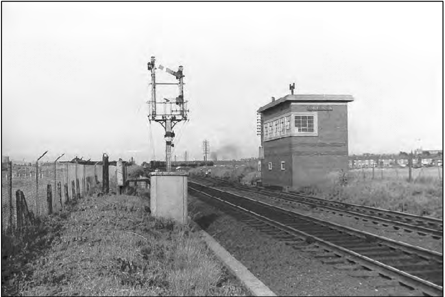
Sankey Junction ARP signal box looking east sometime after 20 May 1968. The signal to the left had controlled Sankey Junction. The signal arms on the right were for the Warrington Central line. The arms for the avoiding line had been to the left but they had been removed when this view was taken as it had gone out of use by this time. Photo by David Lennon
