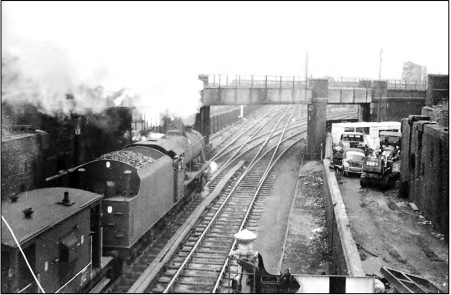
The site of Ann Street Halt looking south towards Widnes Dock Junction seen in the early months of 1967. The bridge abutment seen in the foreground was part of the GR/MR Joint line which passed over Ann Street Halt. Photo by Richard Mercer
