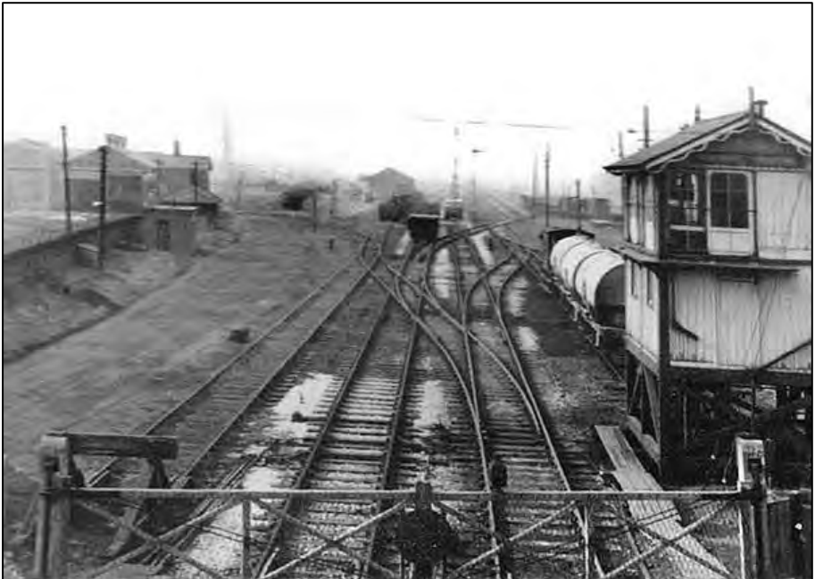
Looking west at Tanhouse Lane yard in 1965 during the period when track lifting was taking place. The main line had been out of use since 6 December 1964 and the signal box had closed on the same day. A crane engaged in the lifting of the up main line can be seen in the distance. Photo by Gordon Howarth
