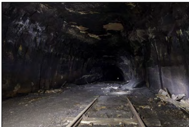
The end of the line. The point inside the Victoria tunnel where the item 41 train brake van came off the rails on Sunday 15 January 1989. After the Waterloo branch had closed in 1973 a stop block had been erected at this point. It was demolished by an earlier runaway and it appears that it was not replaced. This view was taken on 7 December 2015. Photo by Chris Iles
