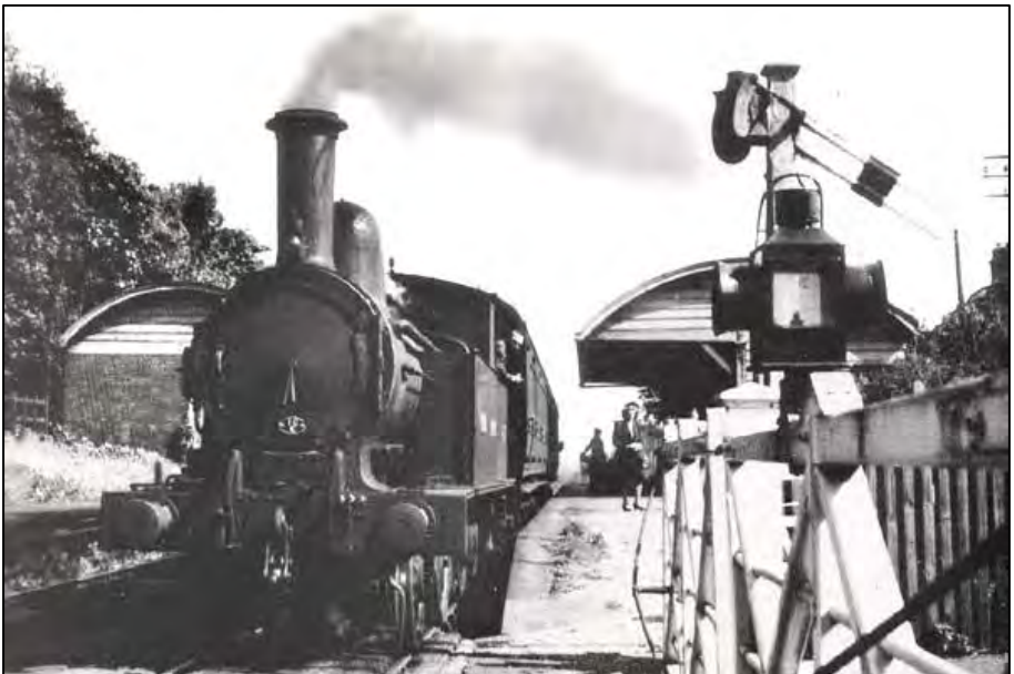
Crank station looking south-east in 1949. Departing from the station in 1949 is a St Helens to Rainford Junction service.
