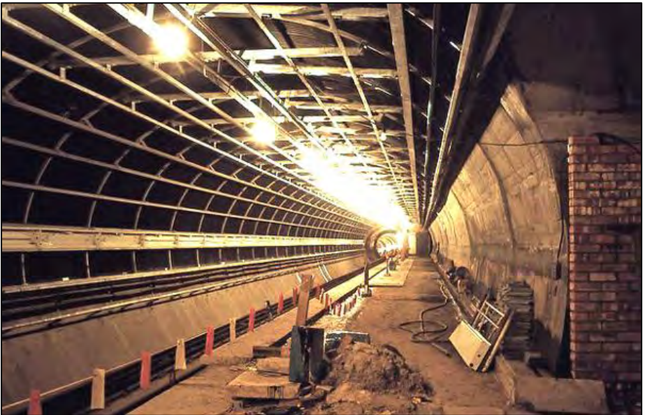
Construction of one the Liverpool Loop platforms in 1975/6.
