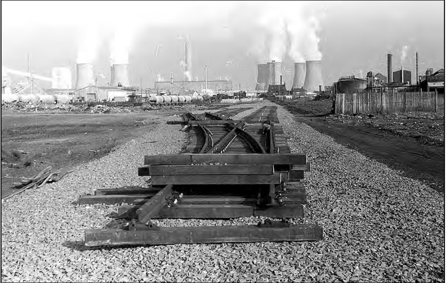
The new sidings at Tanhouse Lane being laid out in February 1982. The old sidings can be seen in the distance with cement wagons standing on them. The Tanhouse Lane goods shed had been located here just to the left of the new points. Photo by Graham Earle
