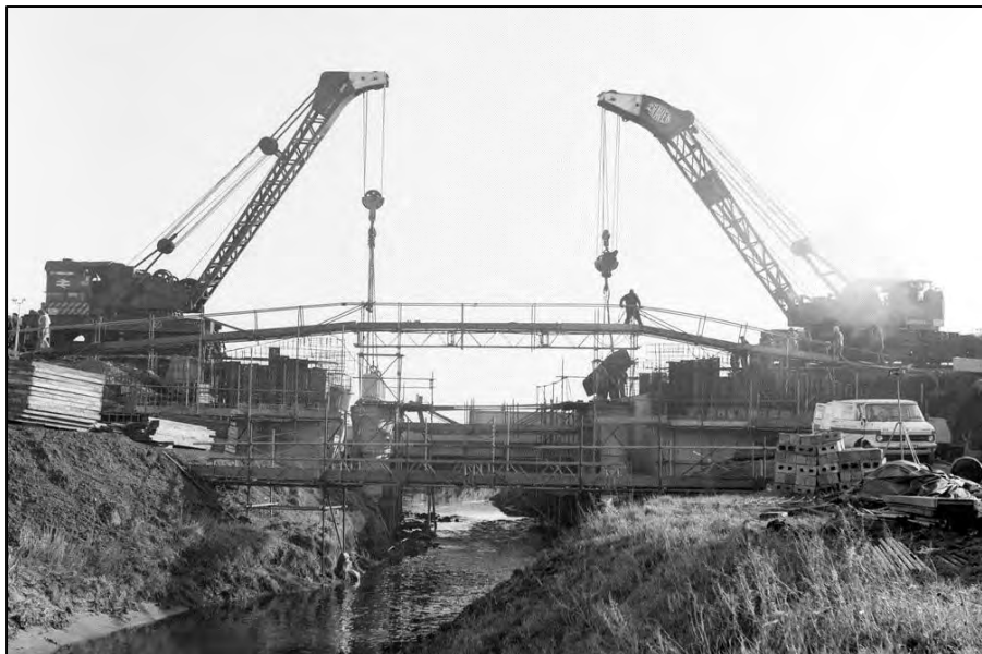
In this view looking south the two steam cranes are seen at work on the replacement of bridge No. 18 on Sunday 13 January 1980. Photo by Tony Foster
