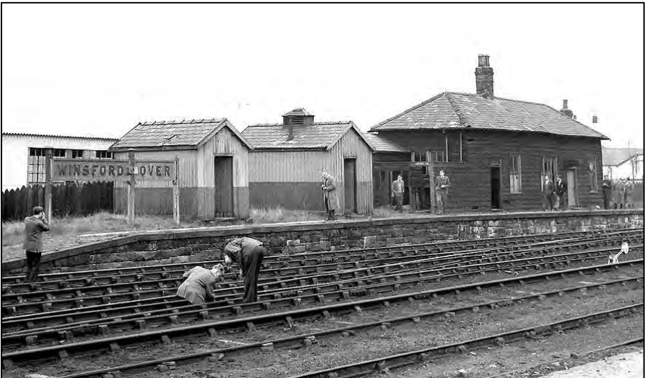
Winsford & Over station on 26 March 1960.
