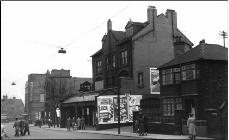
Dingle station seen from street level on 10 April 1955. Photo by D J Norton
