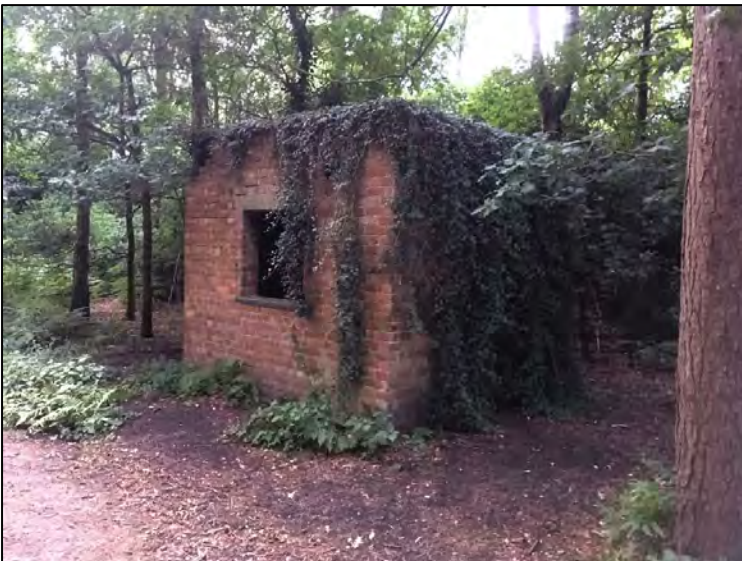
A brick and concrete plate layers hut possibly dating from the 1940s can still be seen towards the northern end of the former CLC Winsford branch. Photo by Paul Wright
