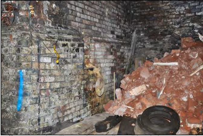
A single buffer attached to the tunnel wall marks the point at which the up line siding at Dingle station came to an end. LOR trains did not have conventional buffers. They had a single buffer centrally positioned at each end of a 3-car unit . Photo by Doug Birmingham
