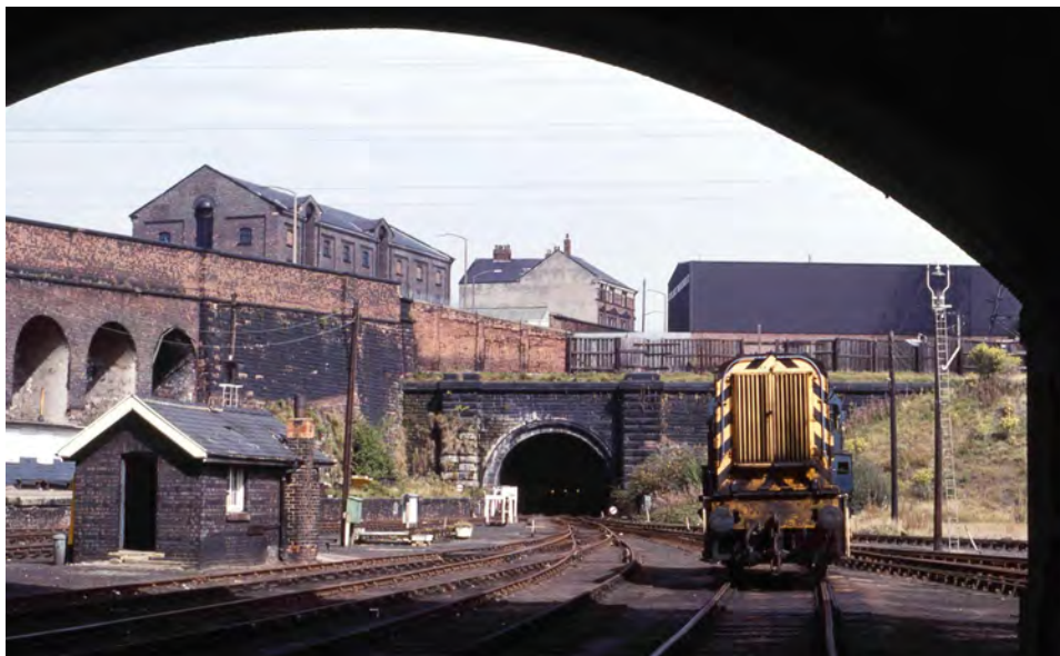
Looking towards the Canada Dock tunnel at Canada Dock Goods Station on 3 September 1982. The heavy engineering features that characterised this station are clearly shown in this view.
