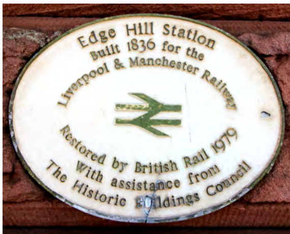
Now in need of its own restoration, the platform wall plate records the 1979 refurbishment of Edge Hill station.
