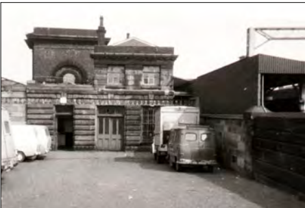
Below : A closer view of the station entrance. The open door at the left was used as the access to the ticket hall. The middle doors were not used.
