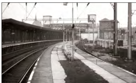
A view of the former L&NWR luggage lift bridge looking towards Lime Street Station at Edge Hill. The two lift towers can be seen. It was as I was walking across the luggage bridge that I found the LM&SR 1932 Rule Book. The Southport Bay can be seen at the right of the photograph.
