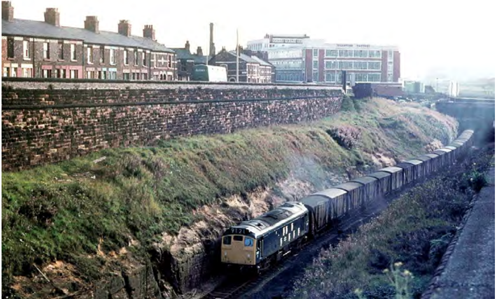
At 16:53 on Friday 7 September 1973 train 9T21 is seen on a Huskisson Dock to Edge Hill trip working . The train is on the Huskisson branch of the CLC North Liverpool Extension Line close to Kirkdale station. It had only just departed from Huskisson. At the head of the train is Sulzer Type 2 locomotive number 7597. This was the era when the former CLC line was in its death throes. By this time the line had become a single track all the way down to Gateacre. A fire had recently occurred at Gateacre signal box and it would be abolished on 26 September 1973 and at the same time the remaining section of line as far as Hunts Cross west Junction was also singled. In July 1975 rail traffic to and from Huskisson ceased. Photo by Alan Roberts
